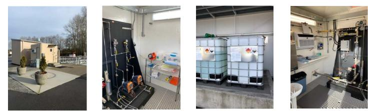
3. The original concern was that PAA might be quickly consumed in the contact chamber – especially in the low flows of summer weather – therefore failing to achieve full disinfection. But after several weeks, it was discovered that a portion of the PAA dose maintained all the way through to outflow. Thus, it did not appear that changing dosing locations would be necessary. The state currently allows Snohomish a no more than 1 ppm residual at final effluent.
